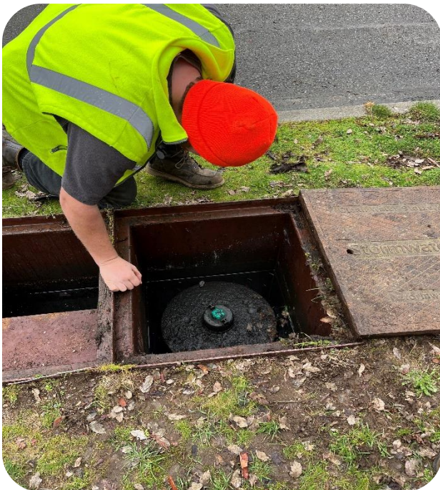
Catchment Basin Inspection Source: Provided by the City of Monroe
