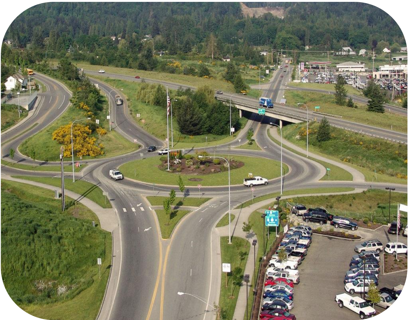
Tester Road Roundabout - Reid Middleton Award
