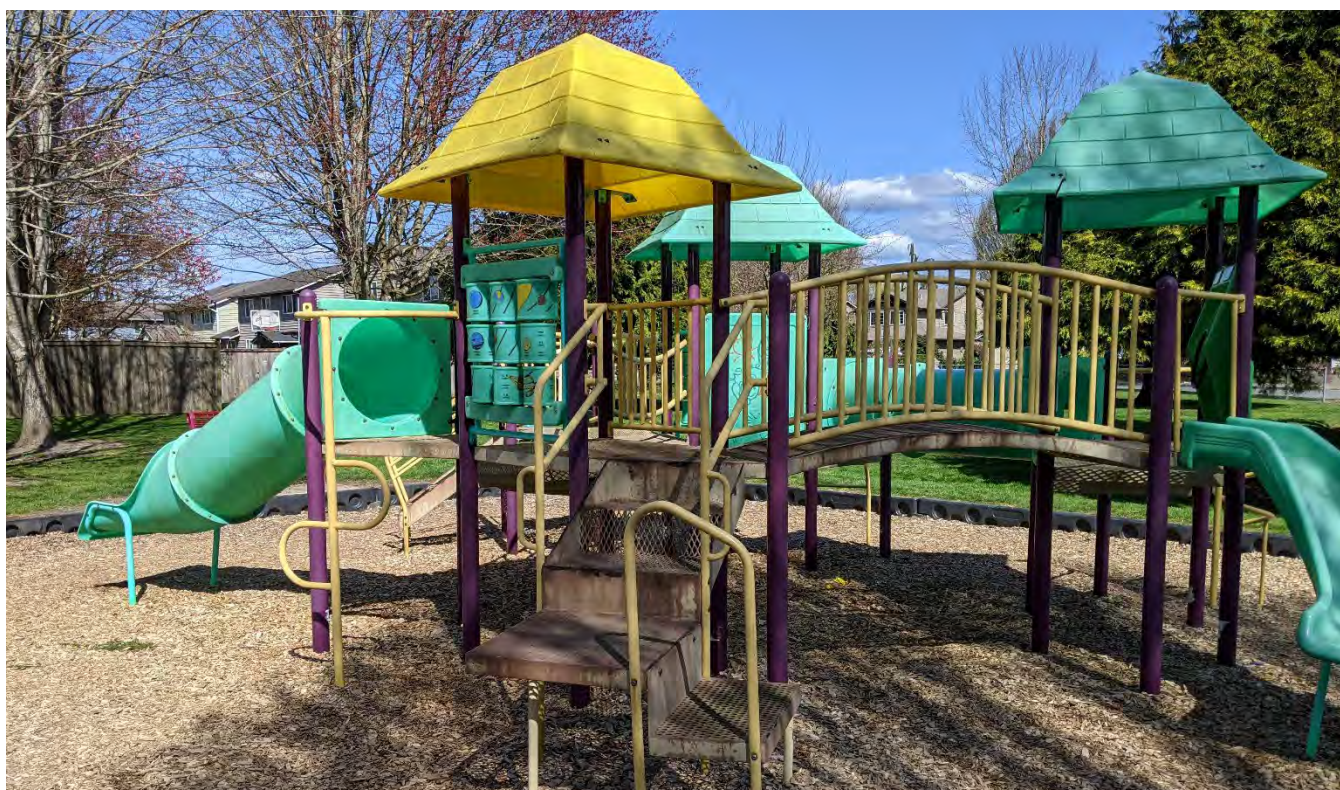
Cedar Grove Park has an example of a playground at the end of its lifecycle that will need to be replaced soon.
