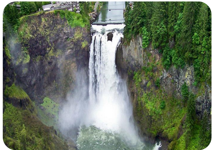
Puget Sound Energy to Cut Carbon Footprint Source: Issaquah Reporter
