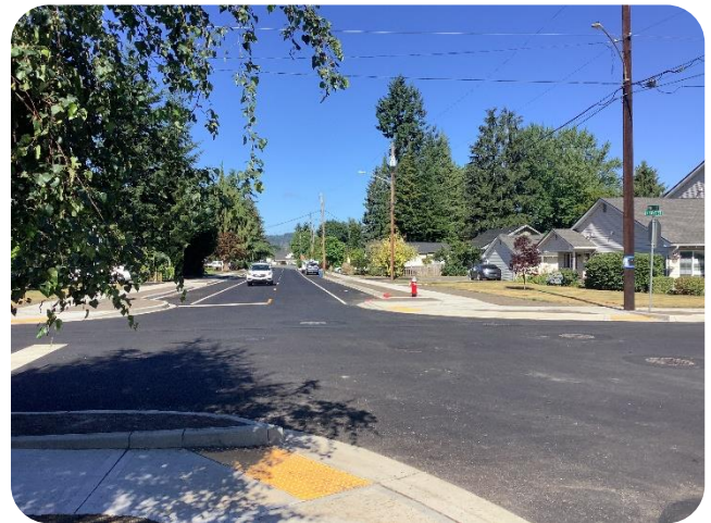
Design and construction in Monroe Source: City of Monroe
