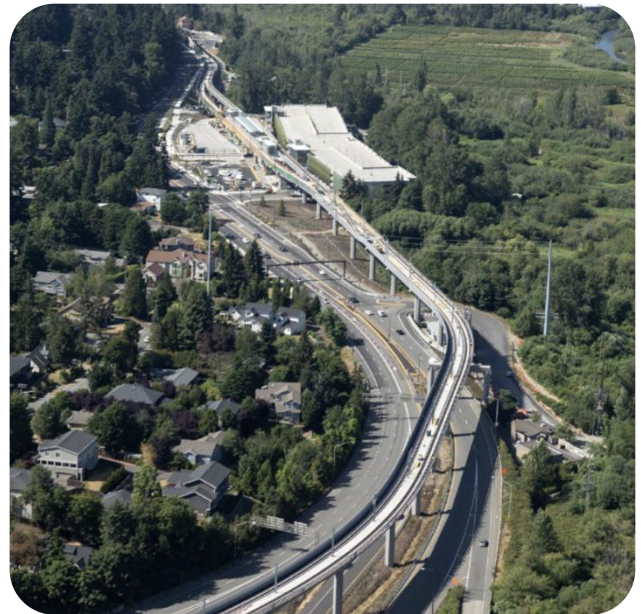
Puget Sound Region Highways Source: Puget Sound Regional Council, 2022
