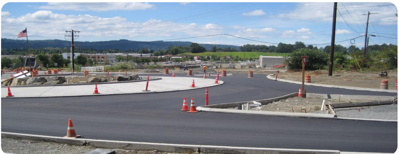
Transportation Improvement Project Source: City of Monroe
